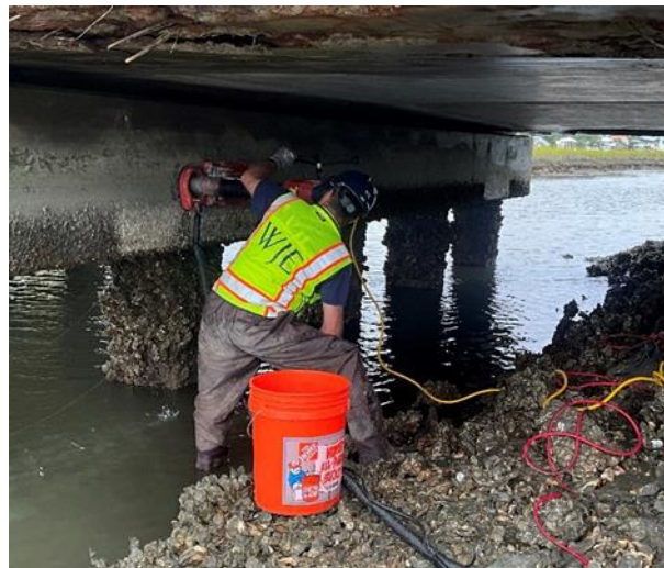
Figure 8. Bent cap 3 core extraction.
