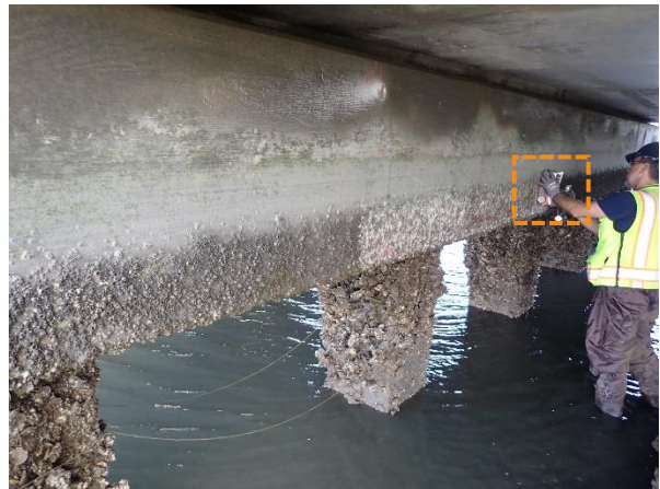
Figure 2. GPR inspection on cleaned face of bent cap 2.
